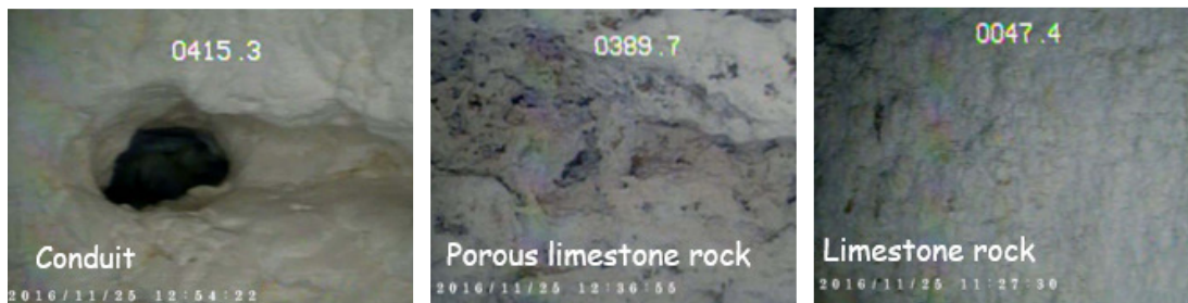
Screenshots from a borehole drilled next to D-22 (low water production)
