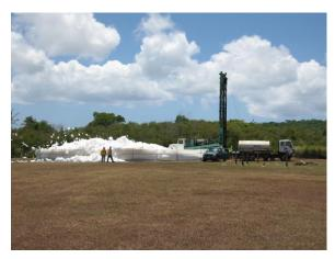
Figure 7. Drilling exploratory well AECOM-11, 21 May 2010. Sites for new water wells should be selected where geologic conditions favor both high water quality and high rates of production.
