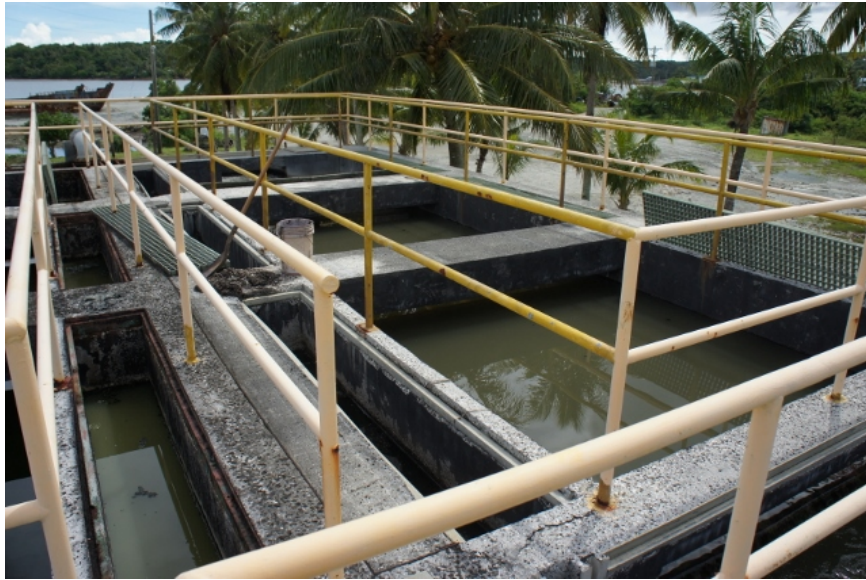
Figure 4. One flow line in the Imhoff tank sewage treatment plant. Image source: author.
