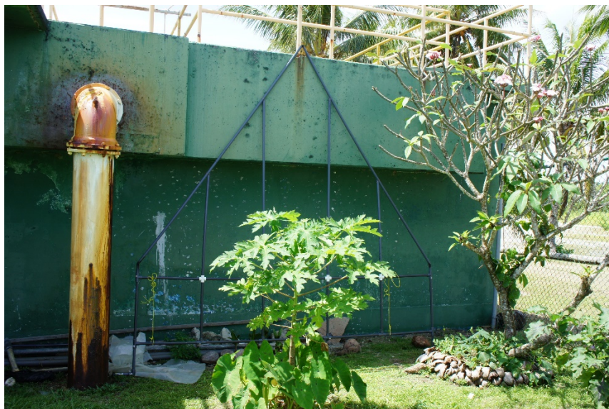
Figure 5. One of six PVC frames (upside-down, behind small papaya tree) used to support mesh material for biofilm attachment. Image source: author.
