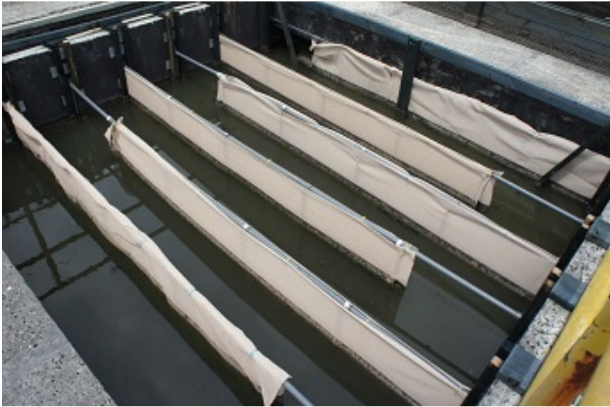
Figure 8. Wastewater flow directed through the biocarrier-frame matrix. Image source: author.
