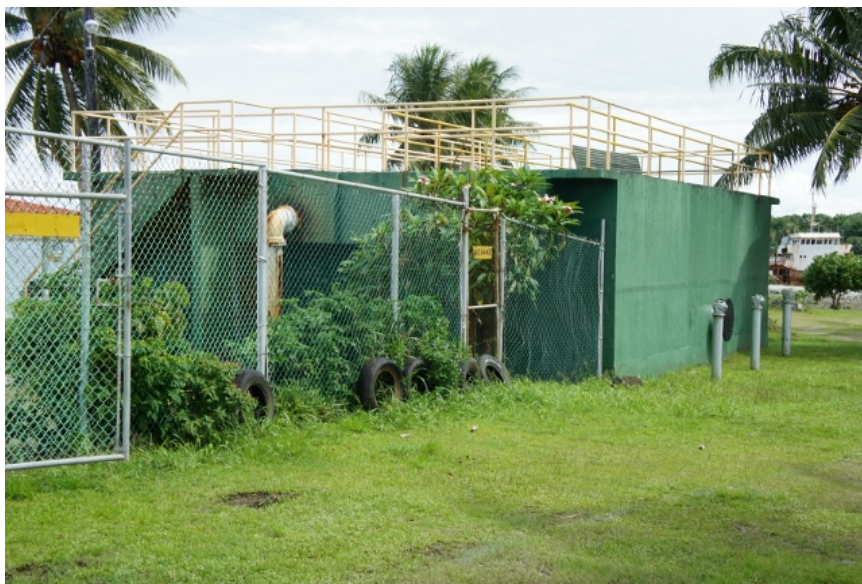
Figure 3. Imhoff tank sewage treatment plant in Colonia, Yap. Image source: author.
