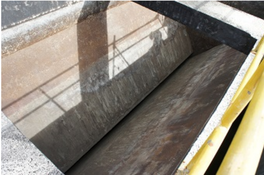
Figure 6. Imhoff tank emptied in preparation for insertion of biocarrier frames. Image source: author.
