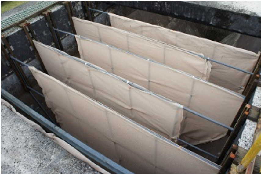
Figure 7. Biocarrier frames inserted in the channel of the Imhoff tank. Image source: author.
