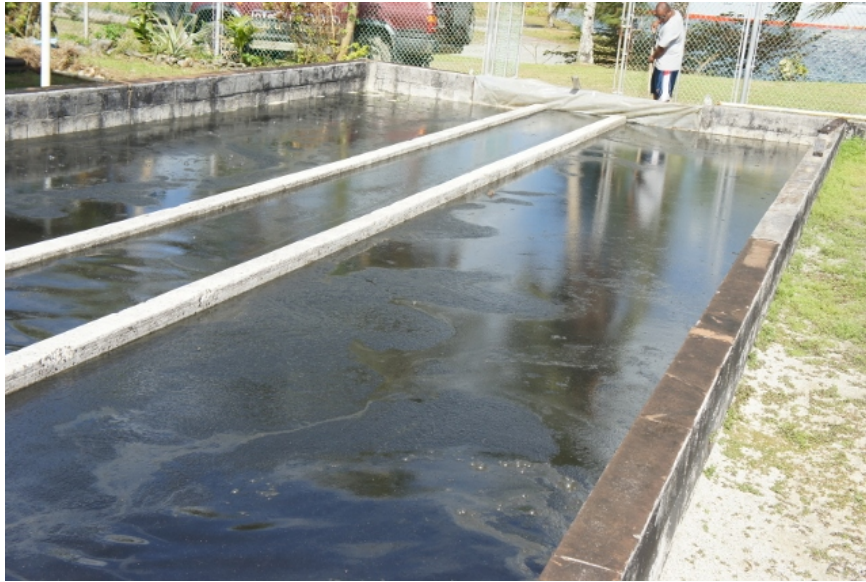
Figure 12. Wet sewage sludge in drying bed at beginning of drying period. Image source: author.
