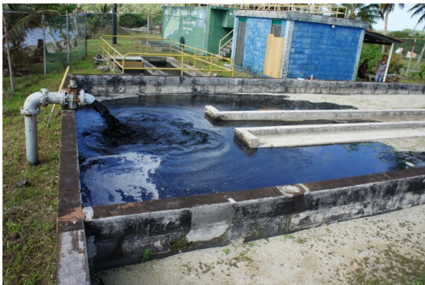
Figure 11. Sewage sludge from Imhoff tank being discharged to a sand drying bed. Image source: author.
