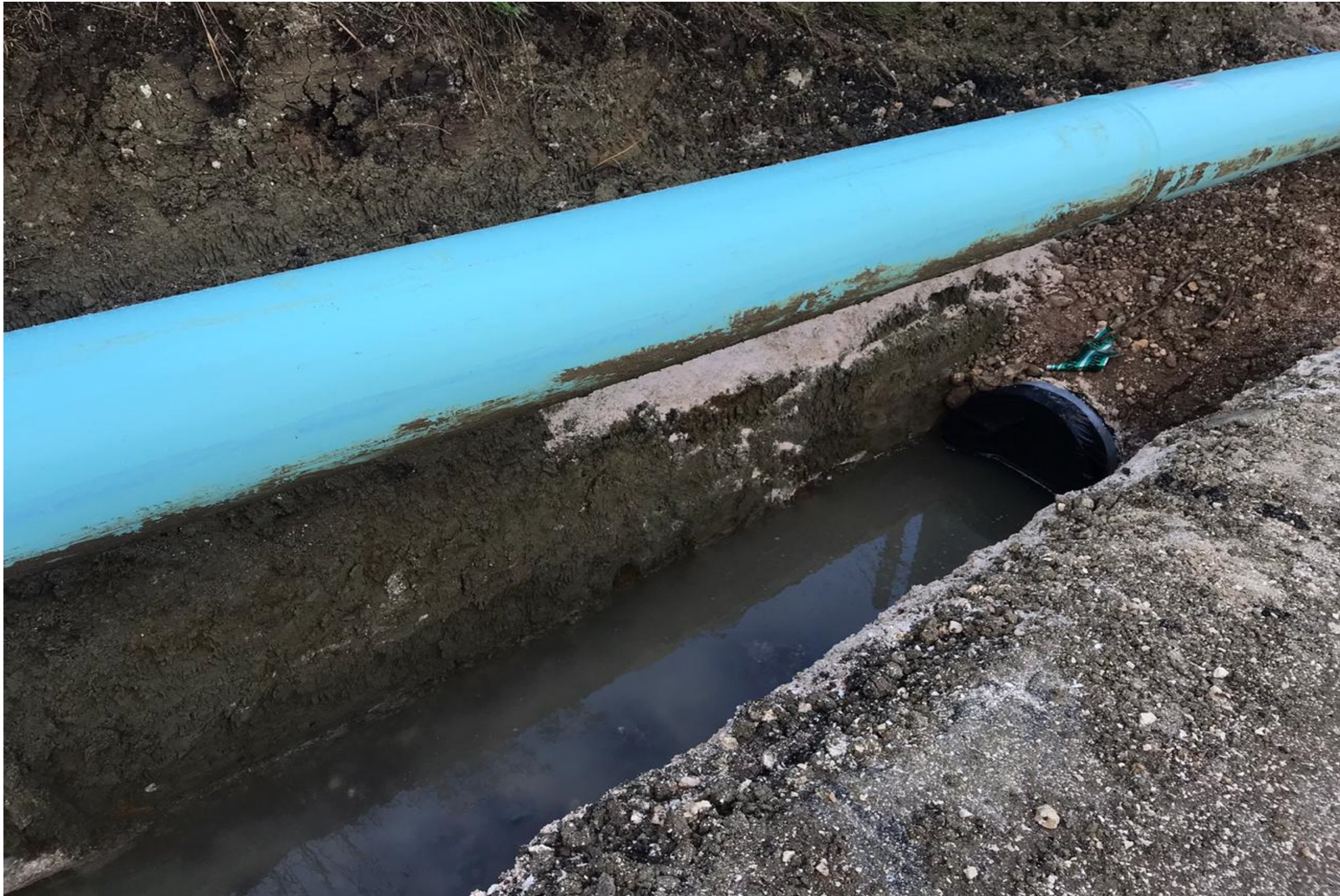
Figure 3.5 (d). Detail of trench cut in the low-permeability Talisay Member, in which the new Navy water main is being installed. Note the standing water in the trench, from recent rainfall.
