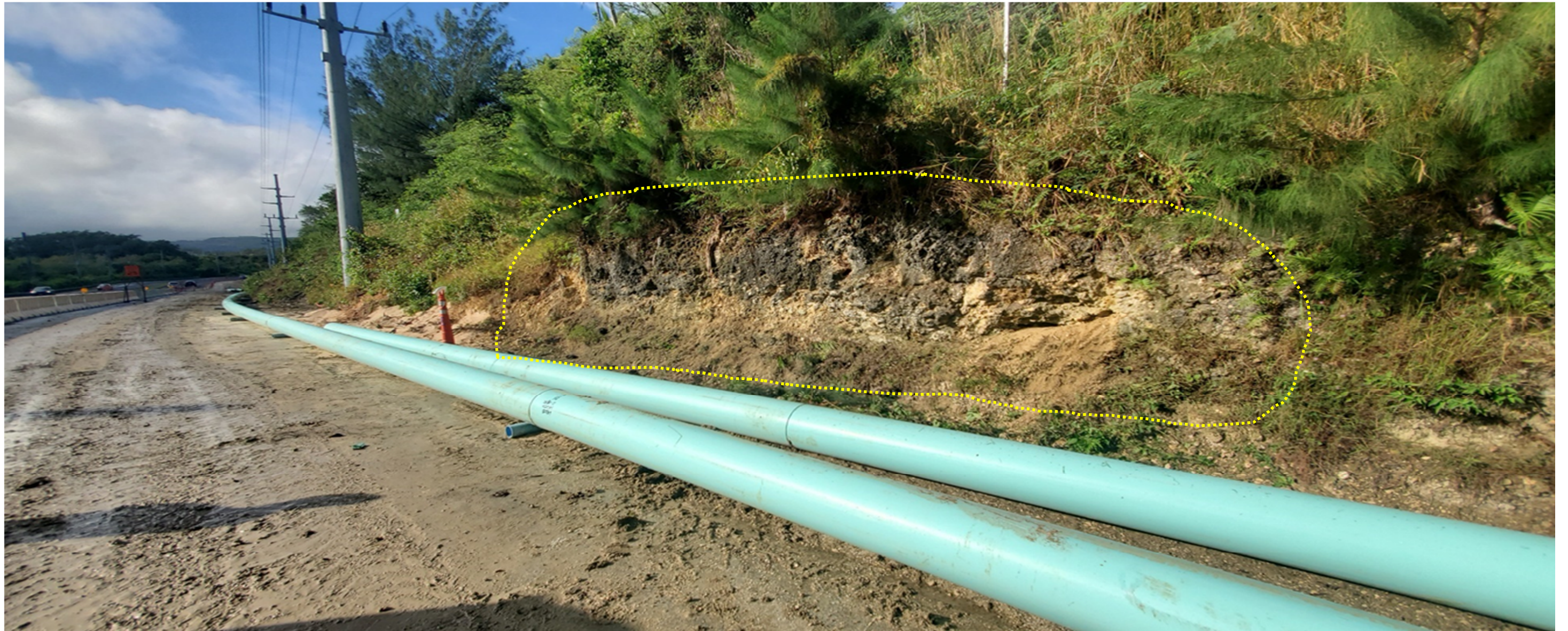
Figure 3.5. (a). Route 1 southbound shoulder showing Alifan-Talisay exposure. Yellow boxed area contains the contact between the overlying Alifan aquifer and the underlying Talisay aquiclude. The teal pipes in the foreground are new 16-in, water main for the Navy water system serving the base.
