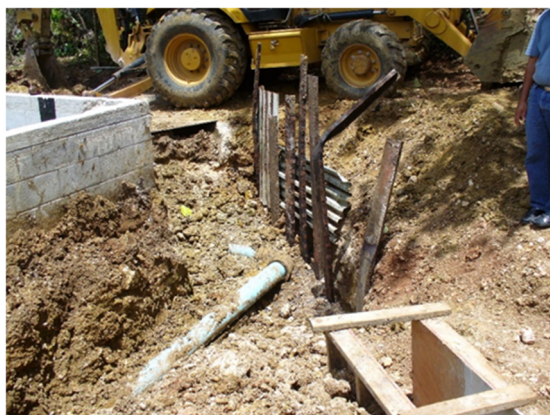
Figure 1.14. Construction of the cutoff wall between Compartment 2 and the booster pump building, 2011. The teal pipe can be seen at the base of the excavation (GWA picture).
