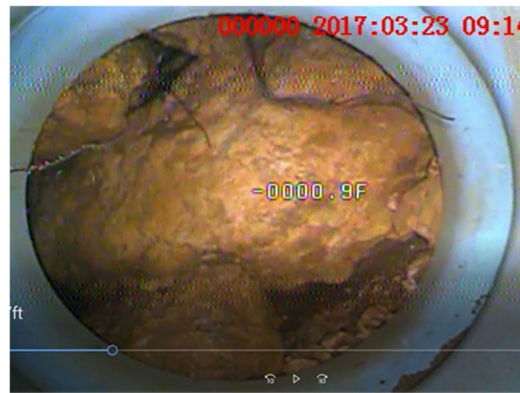
Figure 1.8. Spring collector pipe terminates against limestone cobbles.
