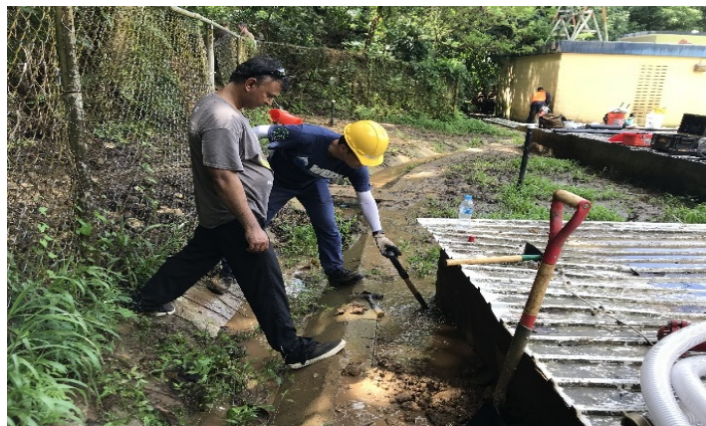
Figure 1.12. Water rising to the surface up along the wall of the spring box, above the spring collector pipe.
