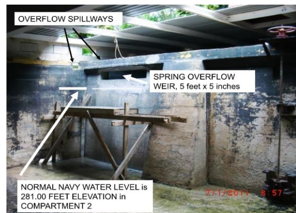
Figure 1.10. Weir between compartments 1 and 2. (GWA picture and measurements.)
