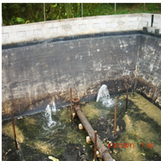
Figure 1.11. Spring water rising up through the floor of compartment 1 during 2011 GWA upgrade work. Photograph provided by GWA.
