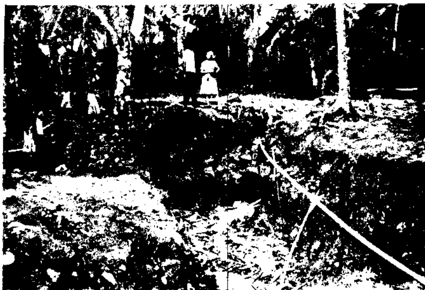
Figure 25. Excavation for sand filter.
