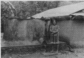
Figure 4. Ferrocement catchment tank with cover (note bent tin gutter).
