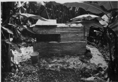
Figure 8. Solar modules temporarily mounted on pump enclosure near Epinup Village.
