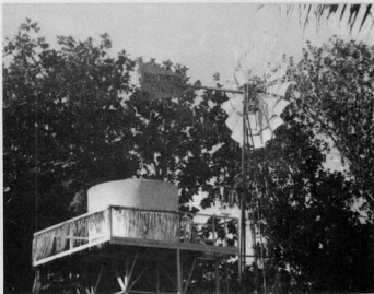
Figure 11. Elevated water tank and windmill at Satawan dispensary.
